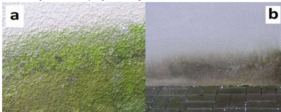
Fig. 3. Parts of the facade adjacent to the ground which the biological film for SEM observation was derived from, a - 30-year-old, non-insulated facade, very porous, b- 14-year-old facade insulated with styrofoam, covered with a thin-layer plaster
