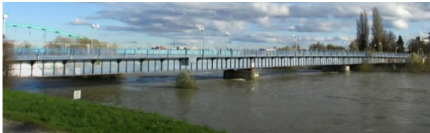
Fig. 1. Road bridge over the Sava River near Zagreb [7]
