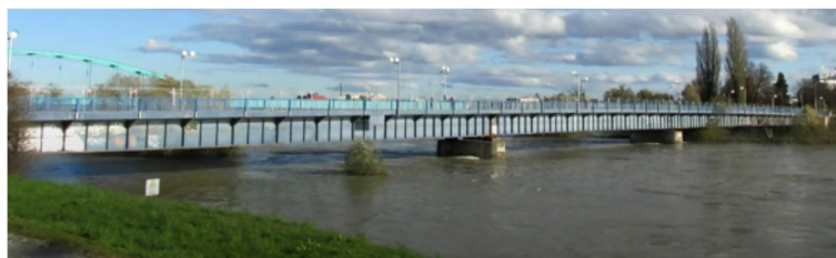
Rys. 1. Most drogowy na Sawie pod Zagrzebiem [7] Fig. 1. Road bridge over the Sava River near Zagreb [7]
