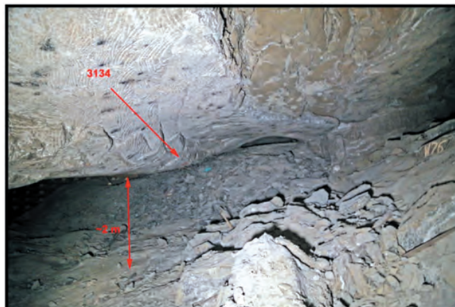
Fig. 4. Baum Chamber. State as of November 2018 [4]
