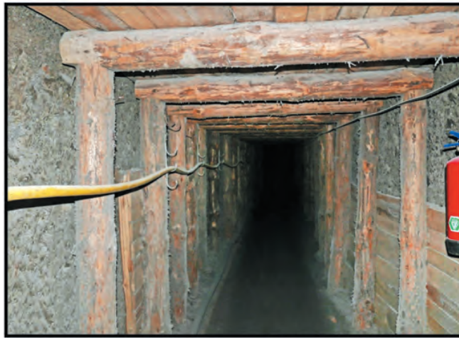
Fig. 5. Schwind Transverse. Area of the planned ventilation shaft. State as of July 2017 [4]
