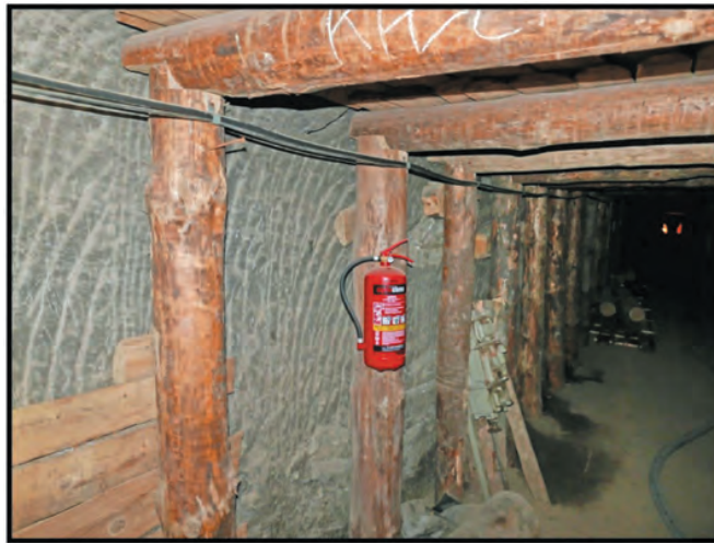
Fig. 3. Baum longitudinal. The area of the planned shaft. Exposure of spizium salts. As of July 2017 [4]
