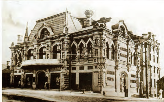
General view and ground floor plan of the Lukyaniv community House . Kiev. 1900-02 Arch. M. Artinov
