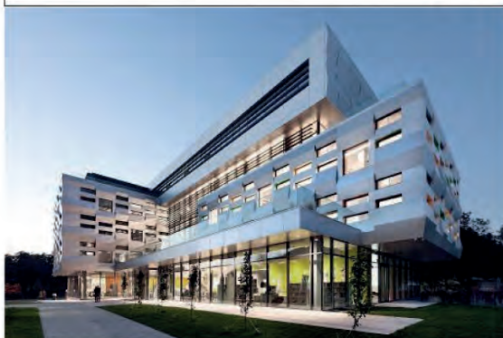
General view and plan diagrams of Andriy Sheptytsky Center. Lviv. 2017 Arch. S. Benish
