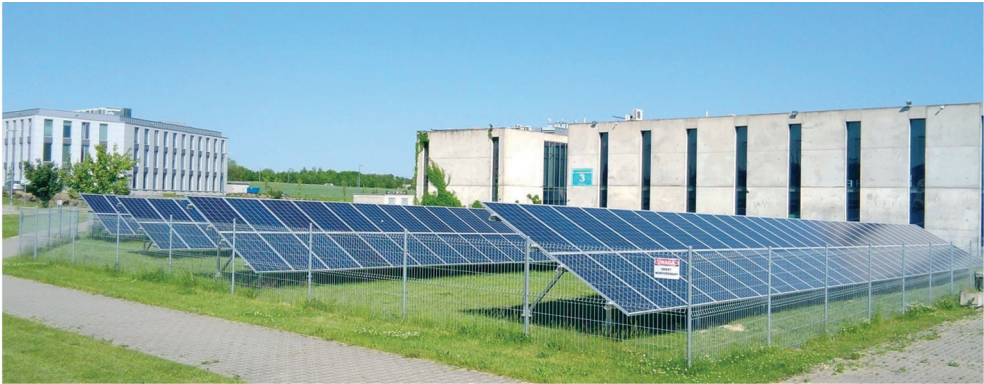
Fig. 1. Appearance of a ground-based photovoltaic system with a peak power of 40 kWp
