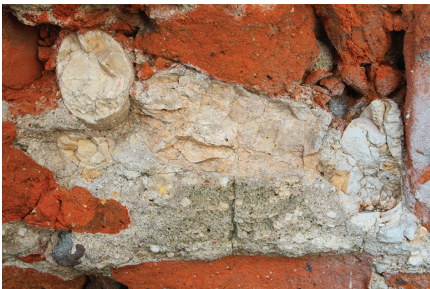
Fig. 4. Castle in Koło. Close-up of the mortar in the joint with visible fragments of calcined limestone (photo by K. Polak, 2020)
