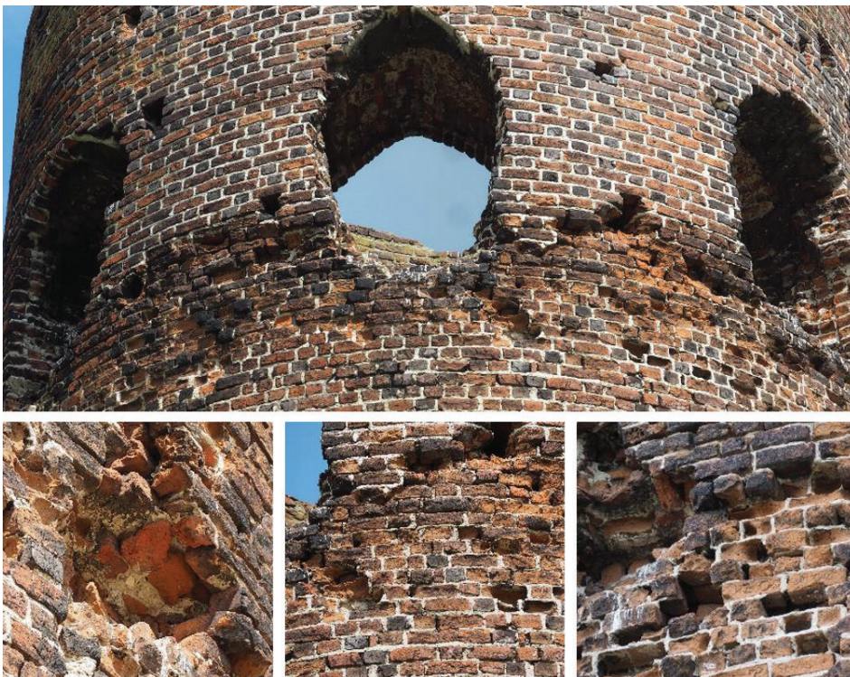
Fig. 8. Castle in Koło. Examples of the state of preservation of the tower walls (photo by K. Polak, 2020)
