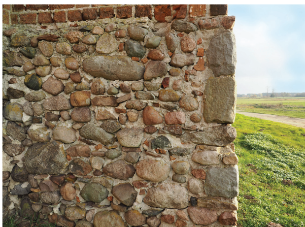
Fig. 2. Castle in Koło. Fragment of a buttress with a restored boulders faced wall with sandstone blocks (photo by K. Polak, 2020)
