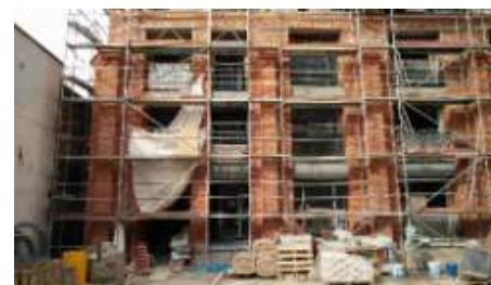
Fig. 5 Built-in historic brick in a newly-built structure 21.03.2017, own archive
