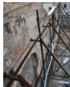
Fig. 10 Protection of walls with steel supporting structure, own archive, 12.10.2015
