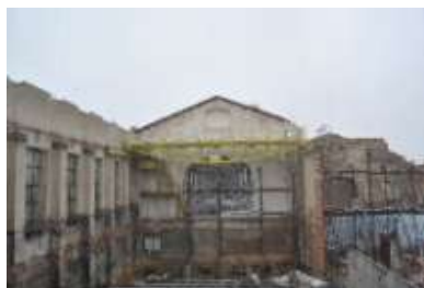
Fig. 4 Old power plant after partial demolition, view of left, 12.10.2015, own archive
