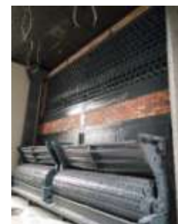
Fig. 8 Two boilers with one drum, steam heater and double grate from Zieleniewski 28.06.2016, own archive
