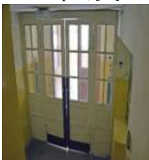
Fig. 6 Paneled wall and double swing doors, Cracow, 2014; source: M. J. Łukacz,
