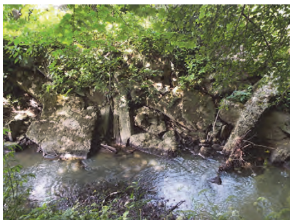
Phot. 3. Bank modification – reinforced from urban debris (RI) (photo L. Borek )
