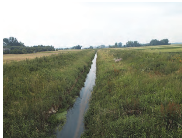
Phot. 10. Uniform bank vegetation structure (U). Resectioned (reprofiled) bank and channel (RS) (photo L. Borek )
