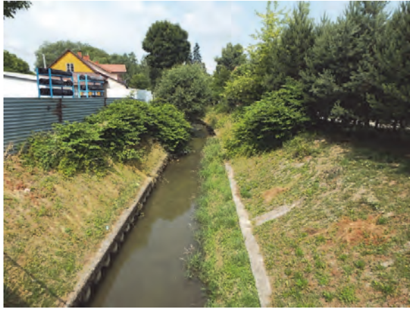
Phot. 5. Reprofiled banks profiles (RS). Uniform (U) and simple (S) vegetation structure. Smooth flow-type (SM). Banks mowing (photo L. Borek )
