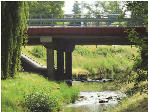
Phot. 7. Major bridge with central piers. Upwelling flow-type (UP) (photo L. Borek )
