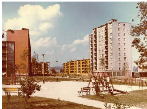
Ill. 11. Green spaces and children playgrounds of mass housing estate Terasa in Košice from the sixties, designed according to principles of modernism.
