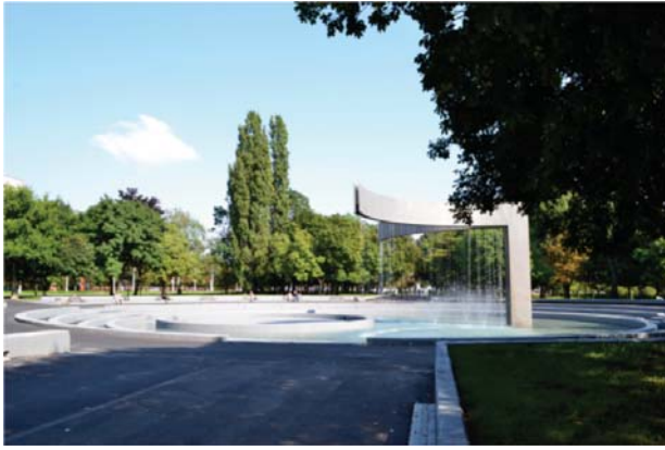
Ill. 12. Park of K. Šmidke (today Park of A. Hlinka) by architect Ferdinand Milučký and landscape architect Alfonz Torma from seventies of the 20 th century represents an outstanding example of the modernist concept of beauty (photo: D. Marcinková, 2014).
