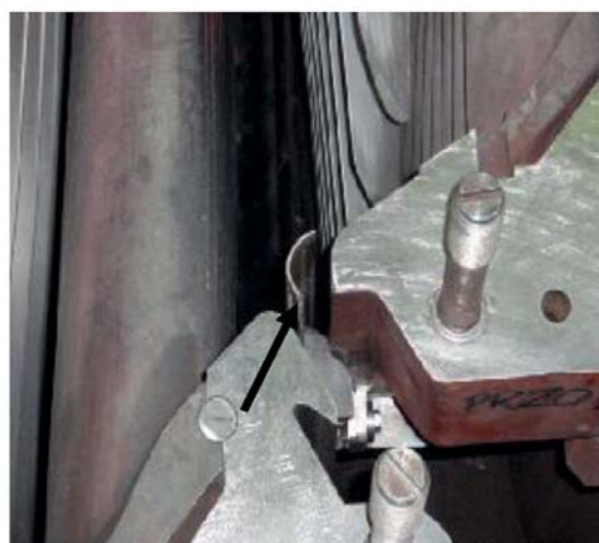
Fig. 13. Photos of the ring installed on stator grips in 225 MW turbine
