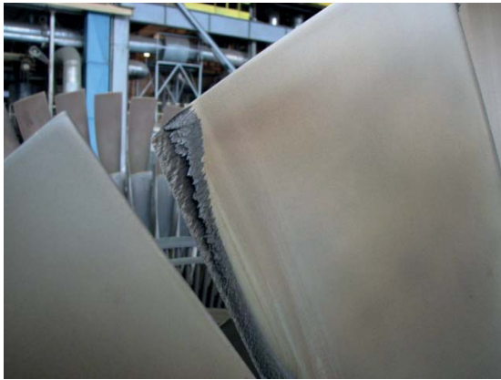
Fig. 4. Leading edge damage patterns observed in the 225 MW turbine last stage rotor blade system
