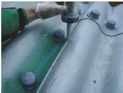
Fig. 3. Filled of structure edge with sealant
