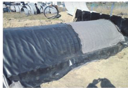
Fig. 18. EPDM geomembrane placed on multi-plate structure
