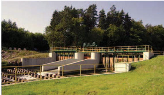
Fig. 1. The dam located next to the hydroelectric power plant
