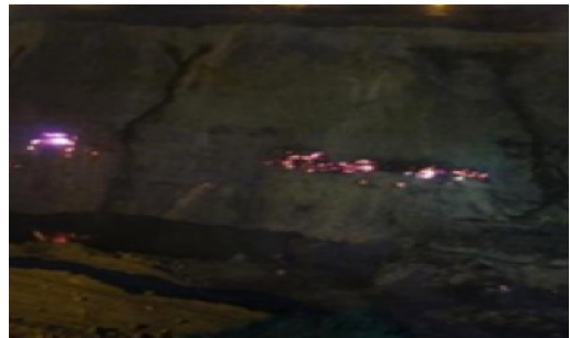
Fig. 3. High wall side near to the coal production area
