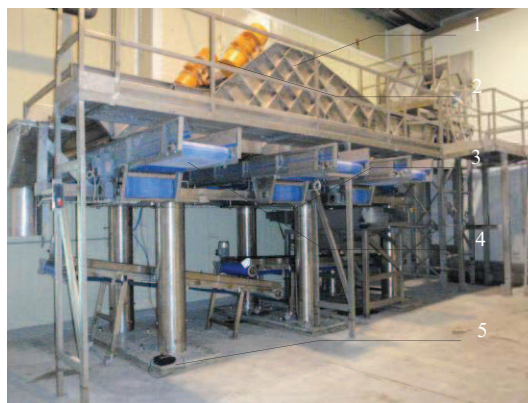
Fig.1. The vibrating screen after modernisation.
