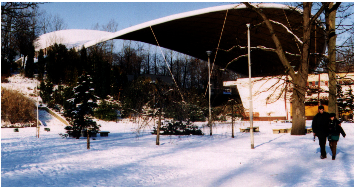
Fig. 1. Suspended roof of the open-air theatre in Koszalin
