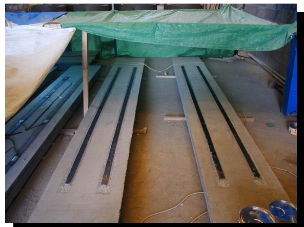
Fig. 6. – strengthening by carbon lamellas.
