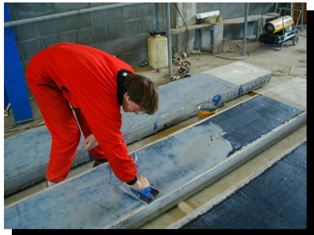
Fig. 8. – strengthening by carbon fabric.
