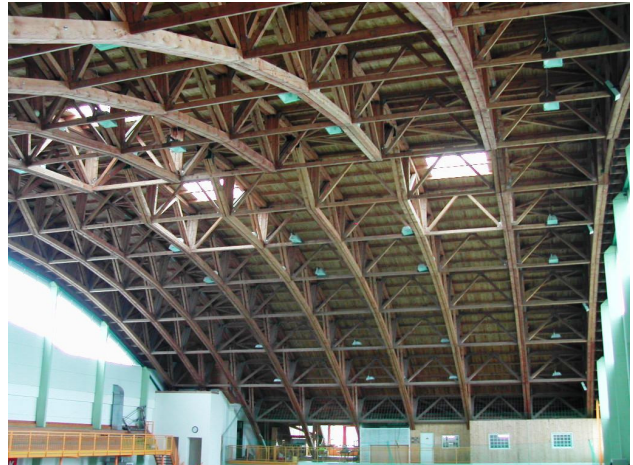
Fig. 4. – roof after its completion.
