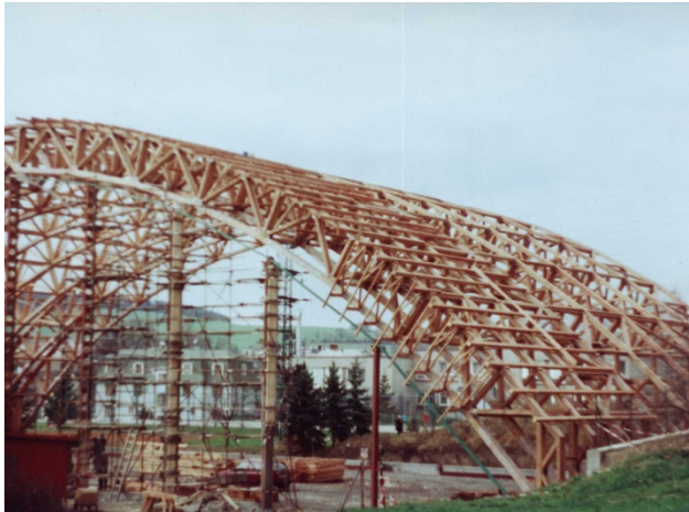
Fig. 3. – hall roof structure in construction phase.
