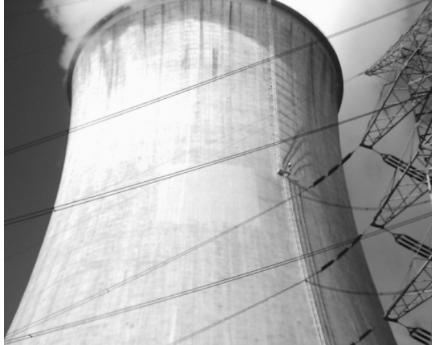
Fig. 9. View of cooling tower.
