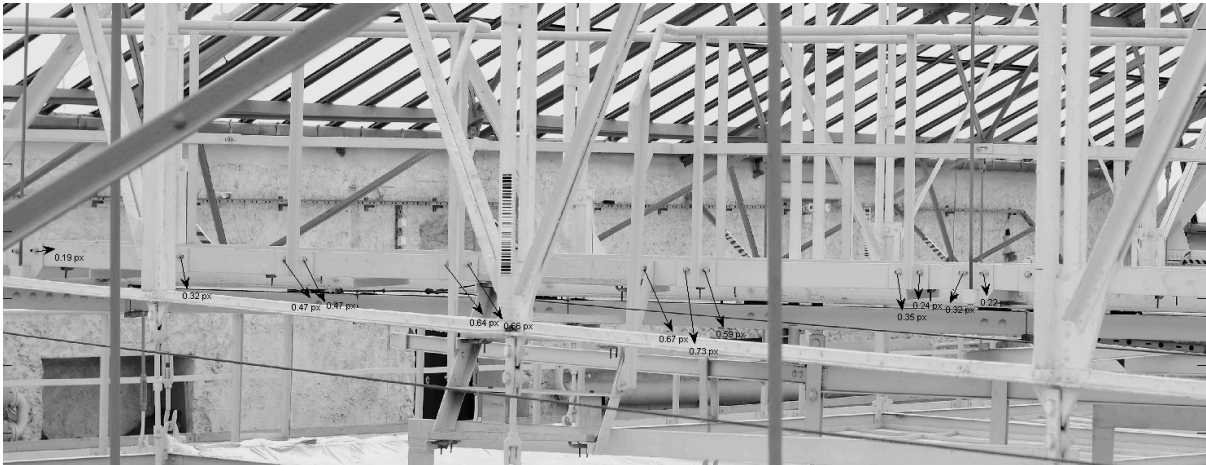
Fig. 7. Result of local registration for selected points on the catwalk. The vectors show calculated shift for selected points. The longest vector is 0.72 pixels what corresponds to around 0.9 mm.
