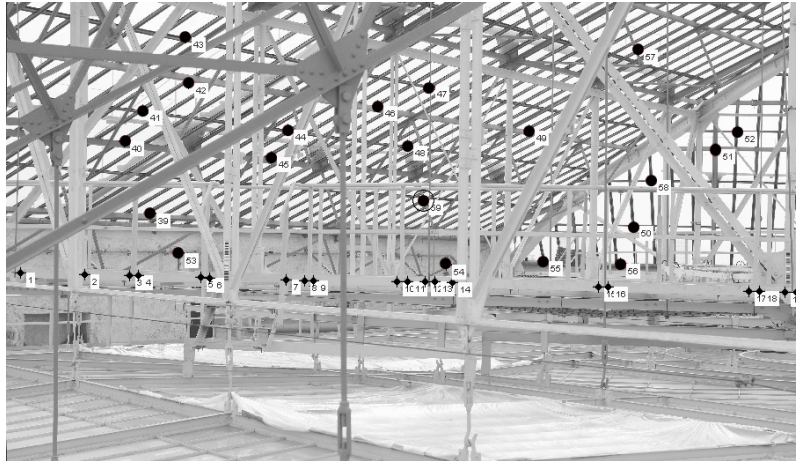
Fig. 3. Control points; black dots – background registration control points; black cross – local points of interest used in deformation estimation.
