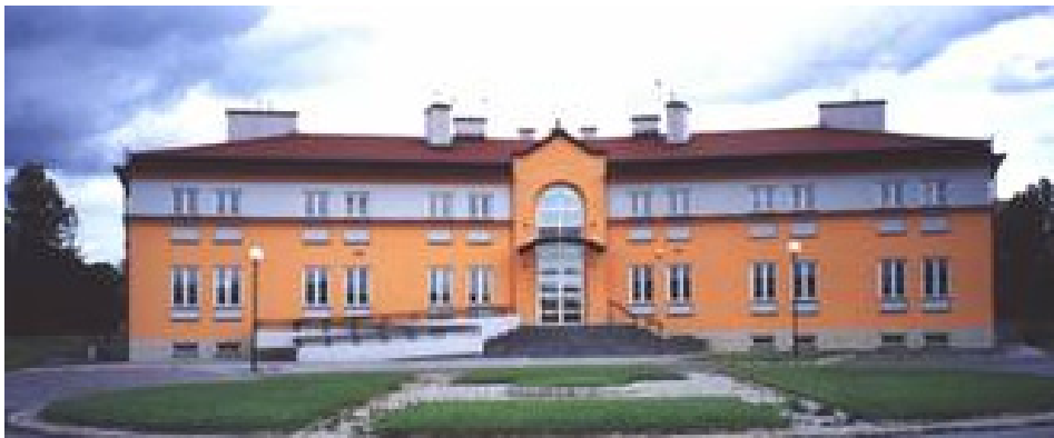
Fig. 3. The new building of the Astro-Geodetical Observatory in Józefosław.
