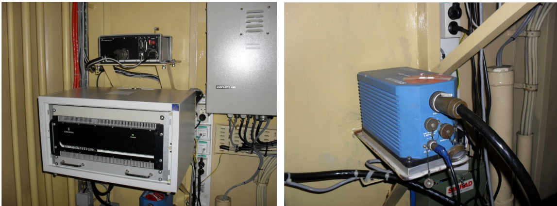
Fig. 3. Multibeam echosounder Simrad EM3000 (down left), singlebeam echosounder Simrad EA400 (top left) and motion sensor Octans (right).
