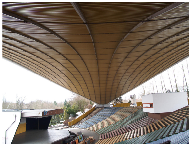
Fig. 1. Suspended roof of the open-air theatre in Koszalin.
