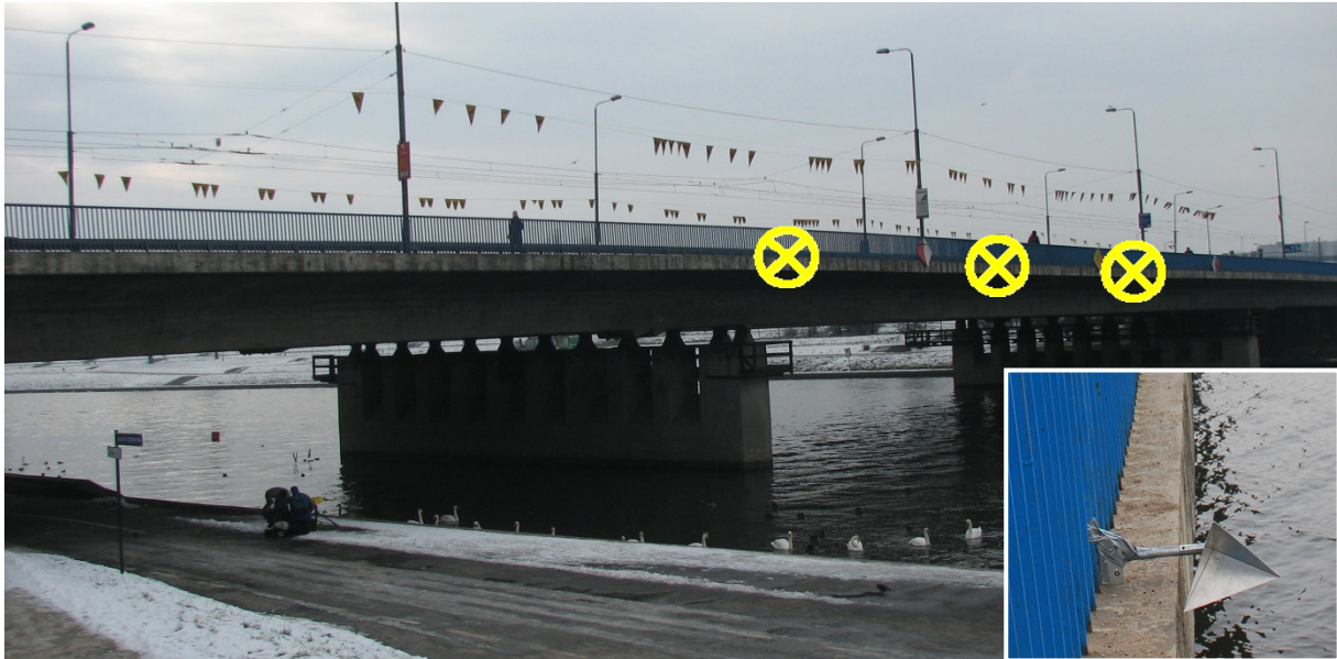
Fig. 7. General view of the Grunwald Bridge and positions of the reflectors.
