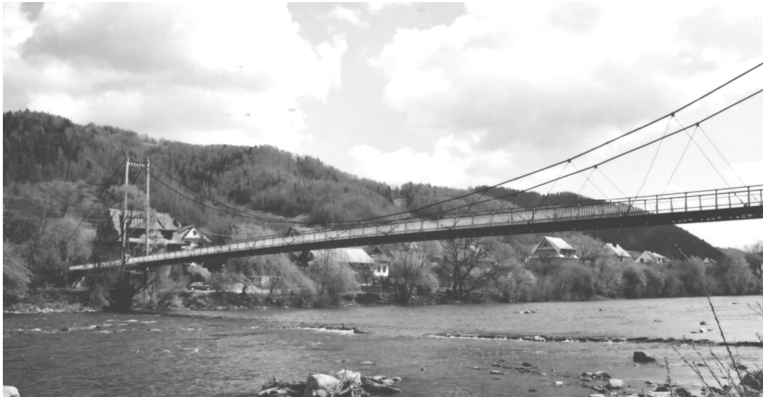
Fig. 1. Tylmanowa footbridge (view from the northern side).
