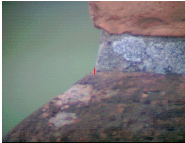
Fig. 2. Image of fotopoint in Total station.
