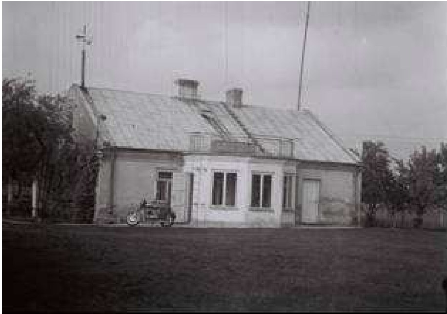
Fig. 3. The first Observatory building.
