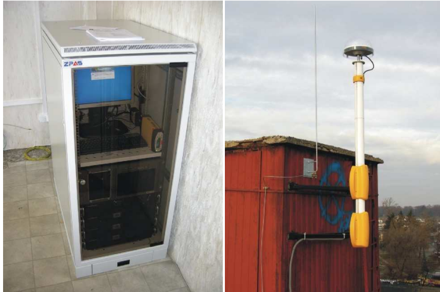
Fig. 1b. ASG-EUPOS BPDŁ station as an example of a GPS/GLONASS station established during the project.
