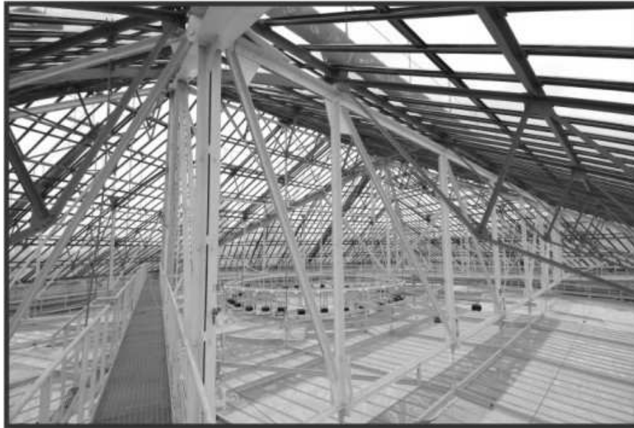
Fig. 1. Roof structure general view
