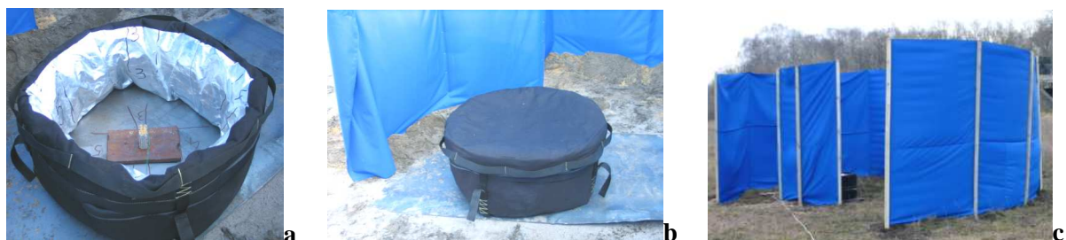
Fig. 7. Cylinder fibrous cover version I view before explosion: a – with TNT slab and balls, without lid; b – with the lid put; c – surrounded with screens of a fabric
