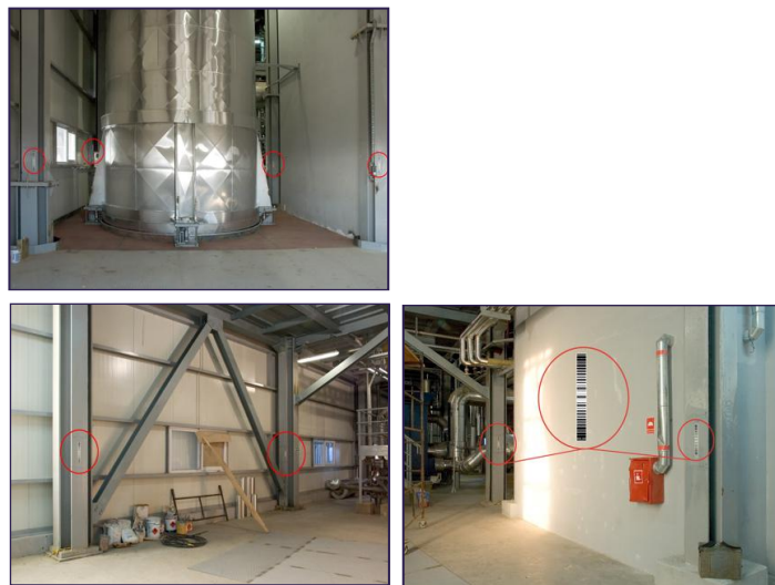
Fig. 3. Control measurement conditions of supporting posts.
