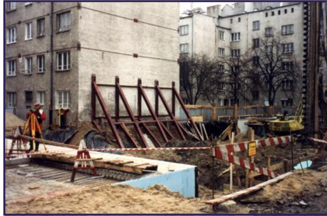
Fig. 5. Trench area - the view of a protective structure.
