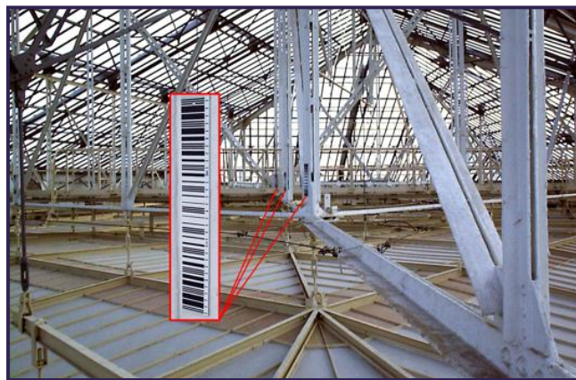
Fig. 4. View of the roof structure over the Main Hall.
