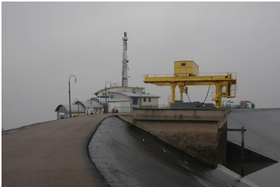
Fig. 7. Dam of the upper Žar reservoir
