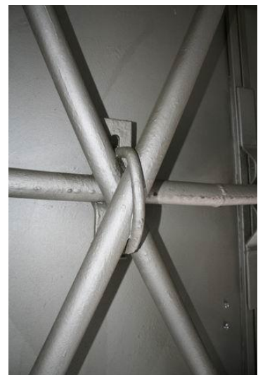
Fig. 4. Connecting yoke.
