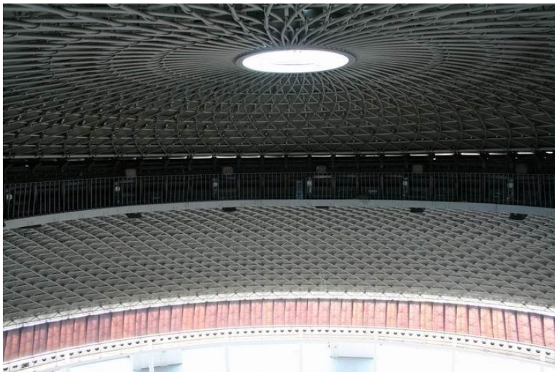
Fig. 3. View of the roof construction.
