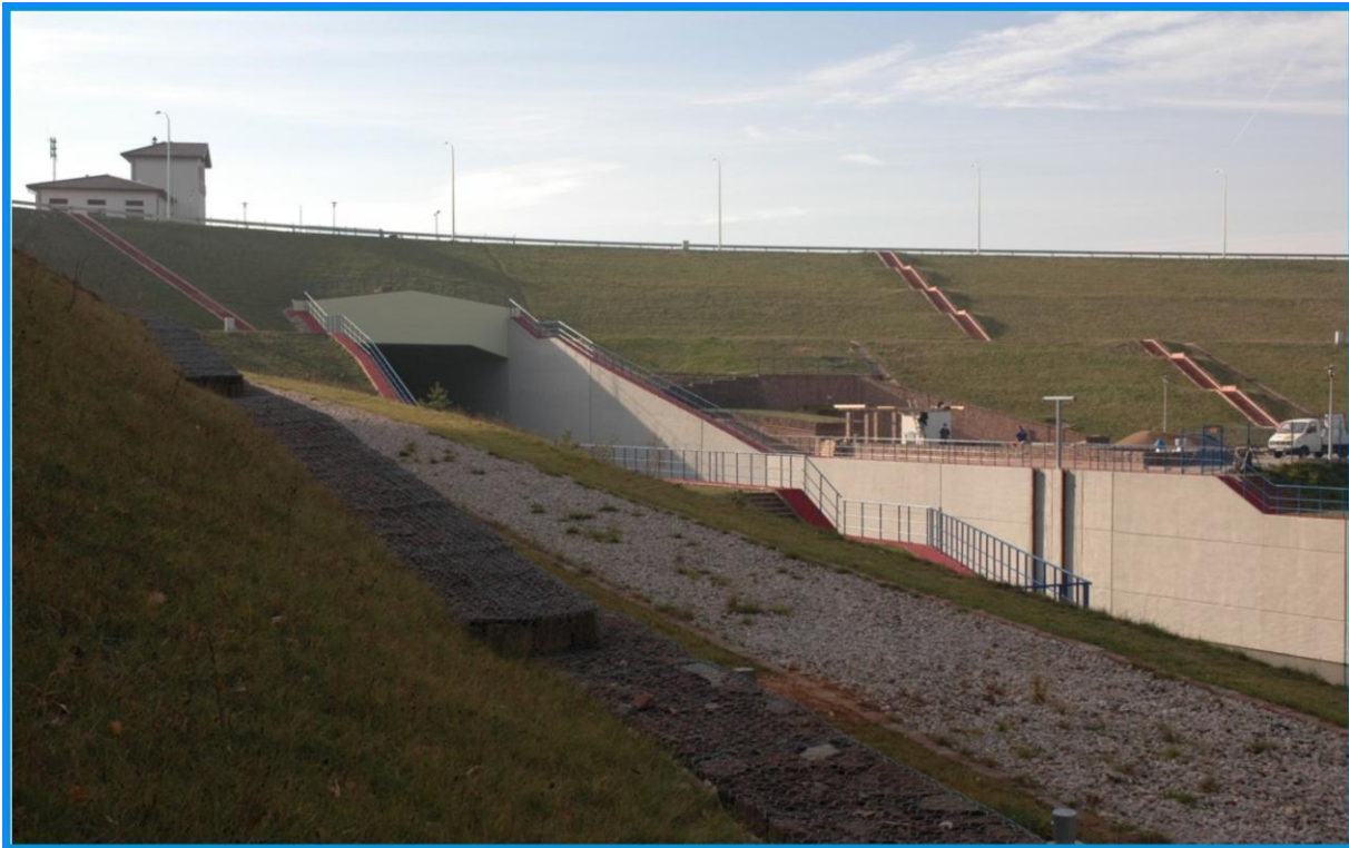
Fig. 2. View of the dam from the lower water level.
