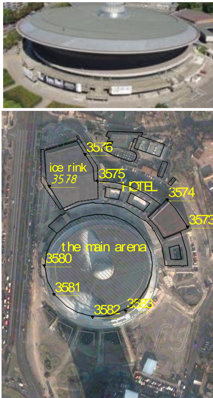
Fig. 1. The aerial views of the study area with localization of leveling benchmarks.
