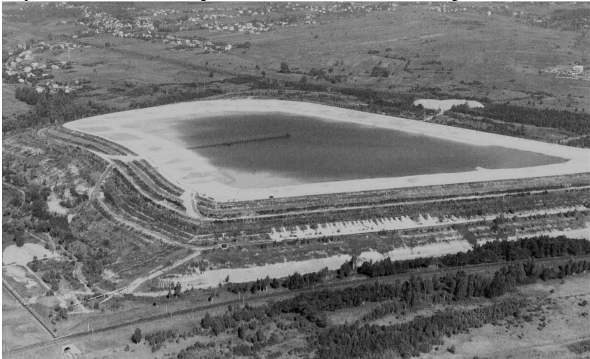
Fig. 1. General view of the landfill.
