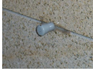
Fig. 2. Controlled bench mark on the Didactic Centre building.
