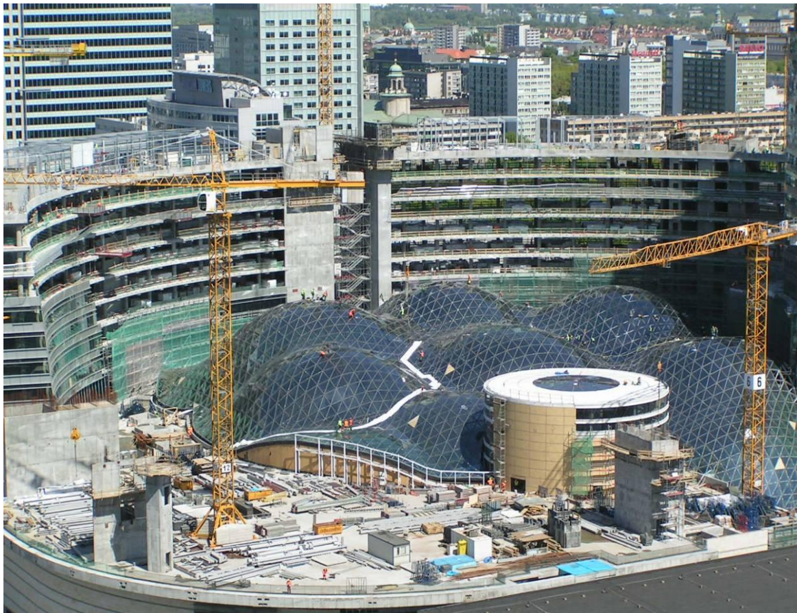
Fig. 2. The Golden Terraces – the general view in the process of construction.
