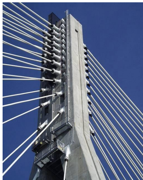
Fig. 4. The Świętokrzyski Bridge - the pylon with rope fastening sleeves.
