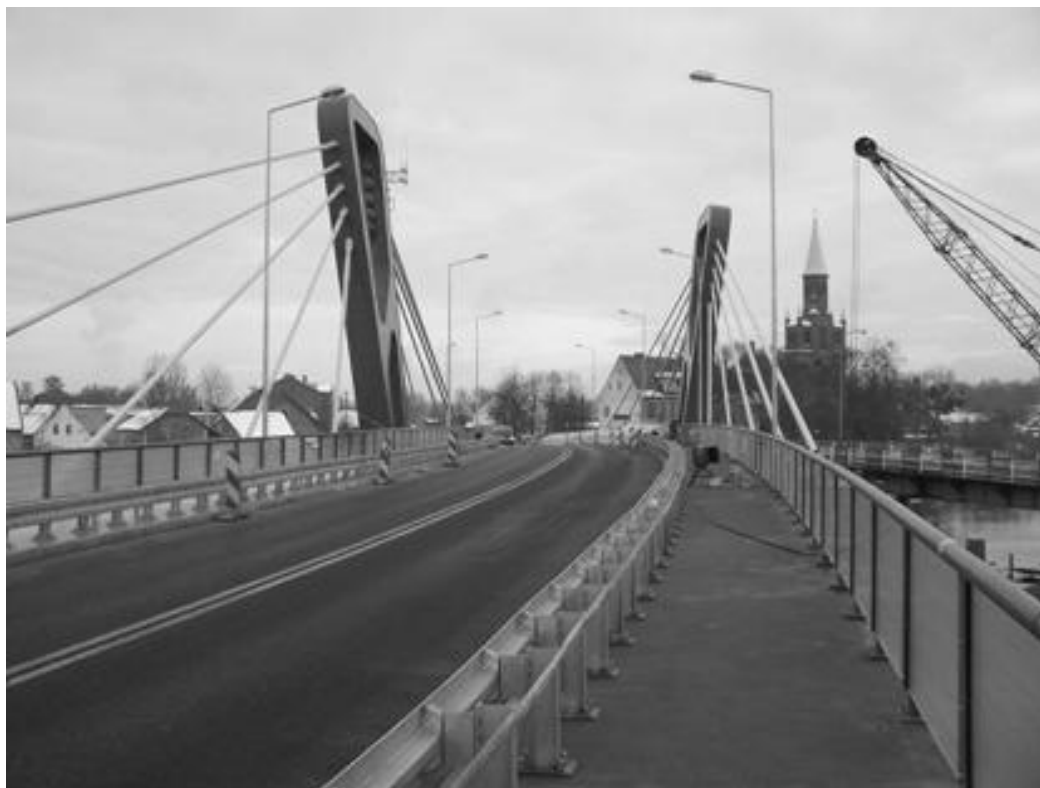
Photo 1. A cable-stayed road bridge, view along the bridge.
