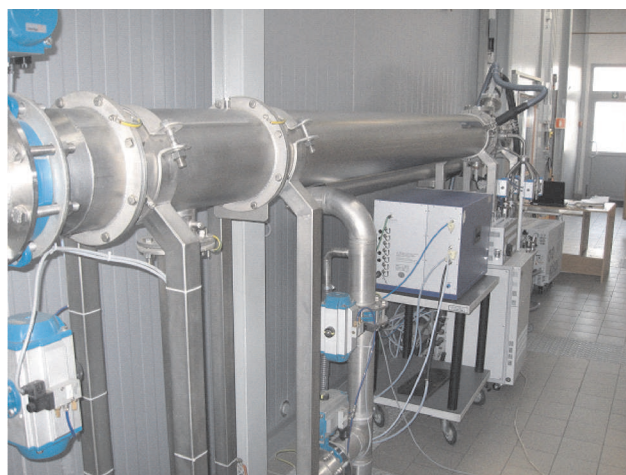
Fig. 9. Dilution tunnel (facing downstream)
