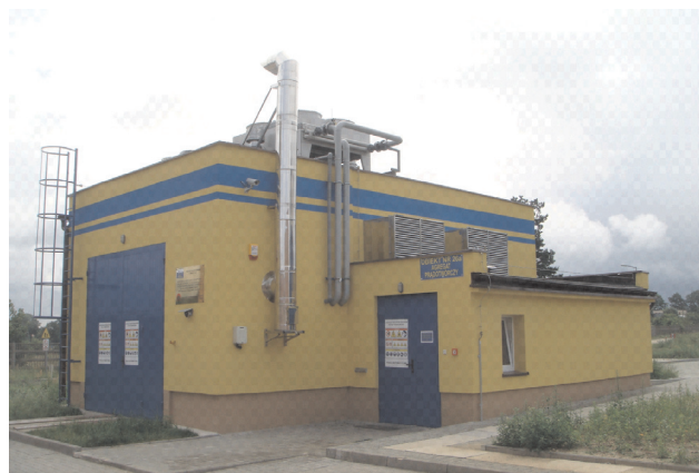
Fig. 1. The thermal-electric power station facility of the WARTA S.A. Waste Treatment Plant in Częstochowa, in which the GE JENBACHER JMS 316 GS-B.LC Engine Biogas Cogeneration Set is installed
