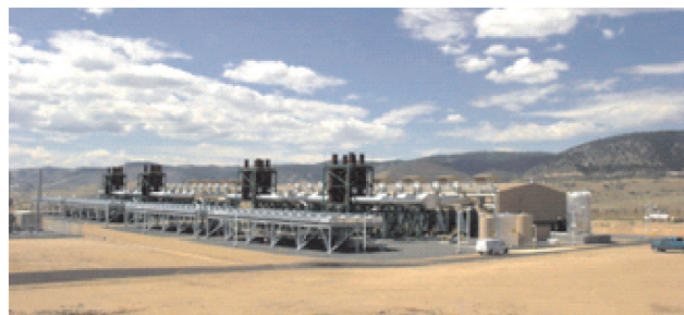
Fig. 5. Plains End power station view
