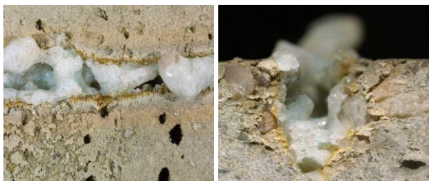
Fig. 6. Concrete sample C30 exposed to 1.6 kW
