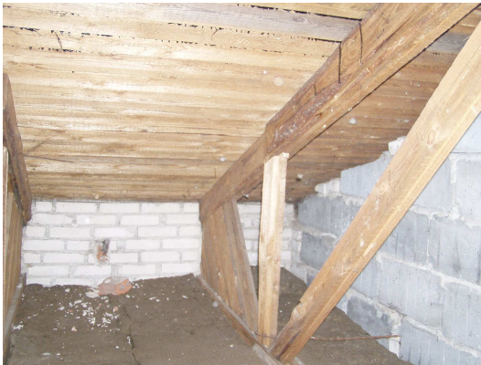
Fig. 2. Investigated pitched roof with non-usable attic.
