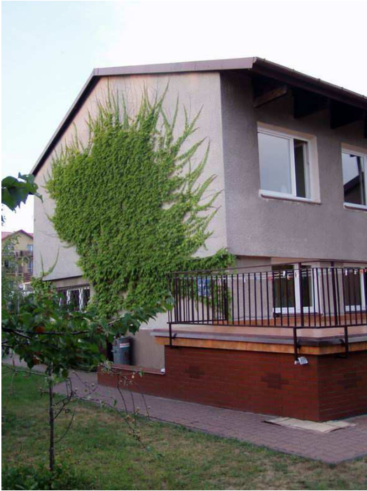
Fig. 1. The investigated building.
