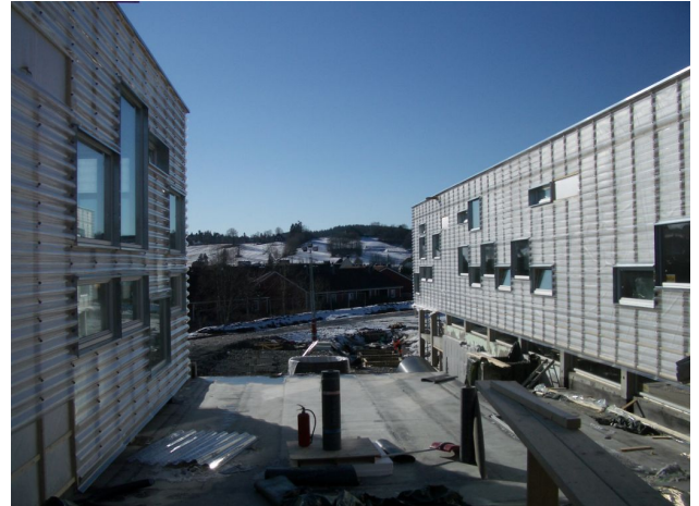
Photo 5. Moniflex walls on two parallel education wings, the nicest view toward the somewhat distant rural landscape.
