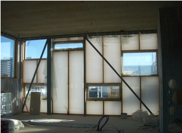
Photo 3. Moniflex wall inside, clear sky and sun.
