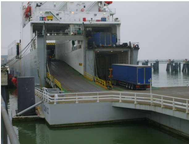
Fig. 3. Pontoon shore ramp linked with ro-ro vessel ramp (Port of Vlissingen)
