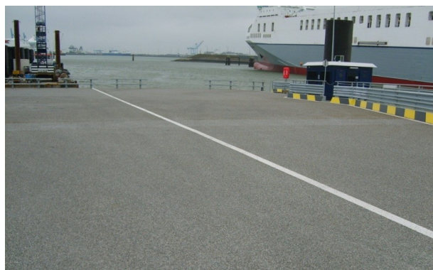
Fig. 7. Pontoon ramp with two loading lines
