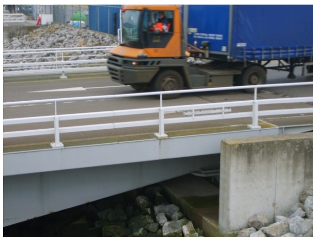
Fig. 6. Loading operation, part of the vehicle located on ramp and part on shore
