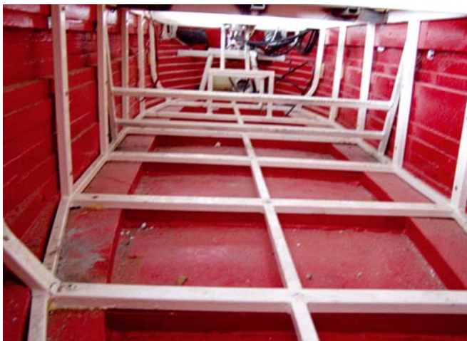
Fig. 2. The steel cage inside the hull. Notice the construction of the hull by red painted slices of wood
