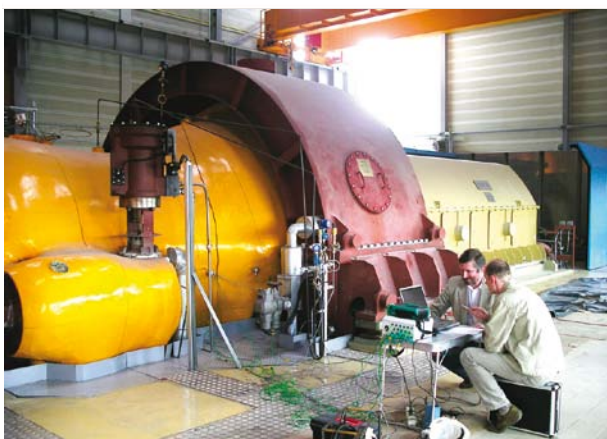
Fig.9 Photo and axial cross-section of 7CK-65 steam turbine set, [4].
