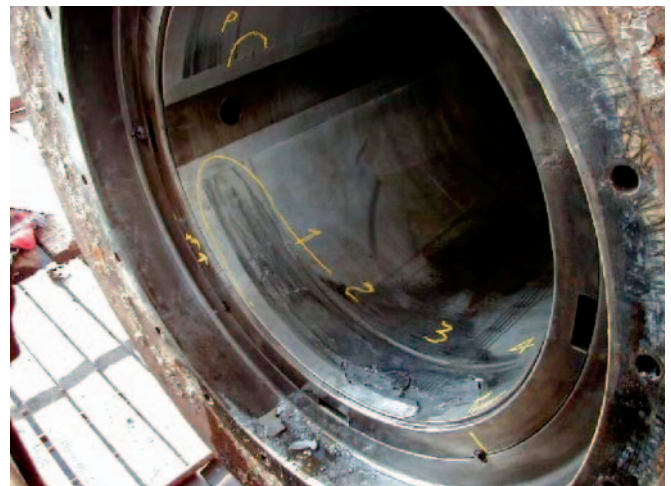
Fig. 7. A white metal bush of oil-lubricated bearing, damaged due to edging
