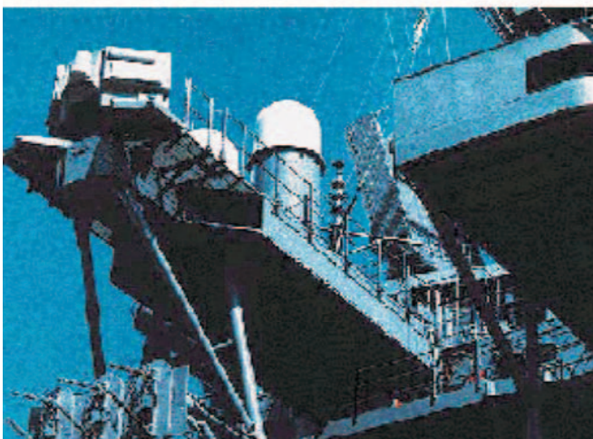
Fig. 1. The aerial platform made of LASCOR panel .
